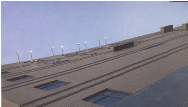
Replacing the signage with LED lighting
