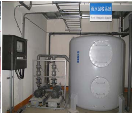
↑ Factories installed with rainwater recycling system
