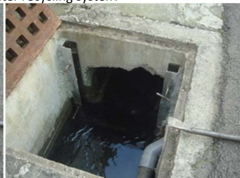
↑ Rainwater gutter installed with water gate for recycle and treatment in stimes of abnormal
