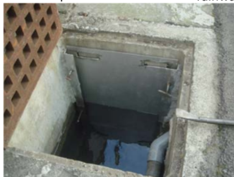
↑ Sludge Storage Zone installed with water division pier
